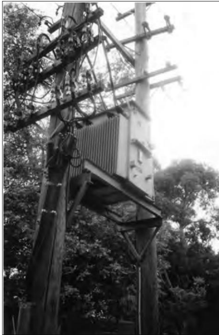
Fig. 12.10 | Transformer pole mounting arrangement: 2-Pole in metropolitan area
