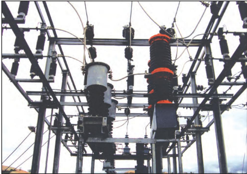
Plate 5 33/11 KV substation: 33 KV MOCBS isolator switches and bus CTS
