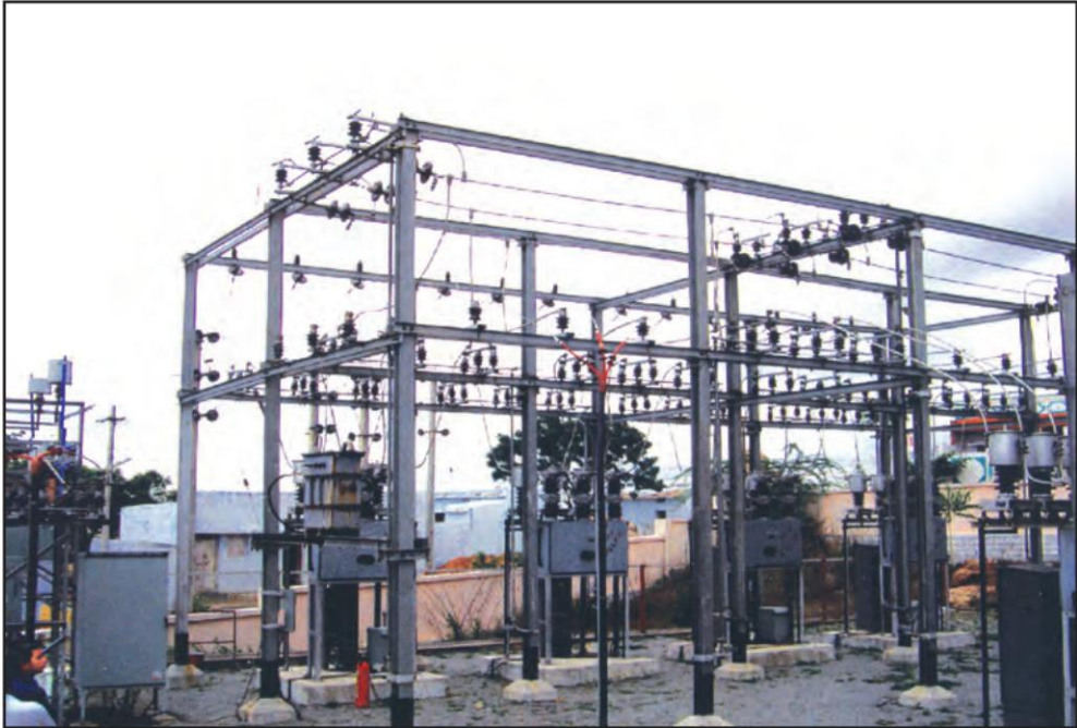
Plate 8 KV bus bars, outgoing feeders with CB & isolators
