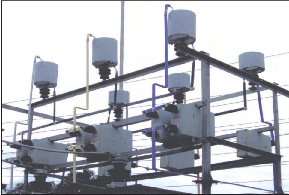
Plate 10 11 KV voltage control capacitor bank with vacuum [BSC on Top]
