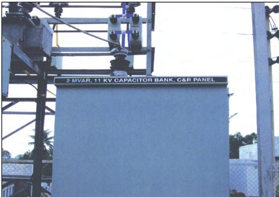
Plate 11 11 KV capacitor bank arrangement with control panel [2 MVAR] [1 phase arrangement of Plate 10]
