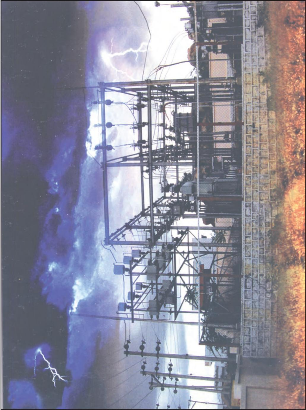
Plate 12 11 KV side of 33/11 KV substation with outgoing feeders [4 numbers & voltage control capacitor bank [Plate 10]
