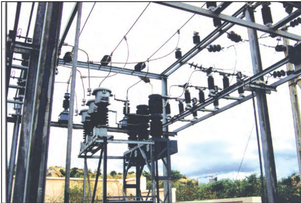
Plate 6 33/11 KV substation bus bar arrangement, air disconnecter switches, lightning arresters, mocers and bus CTS
