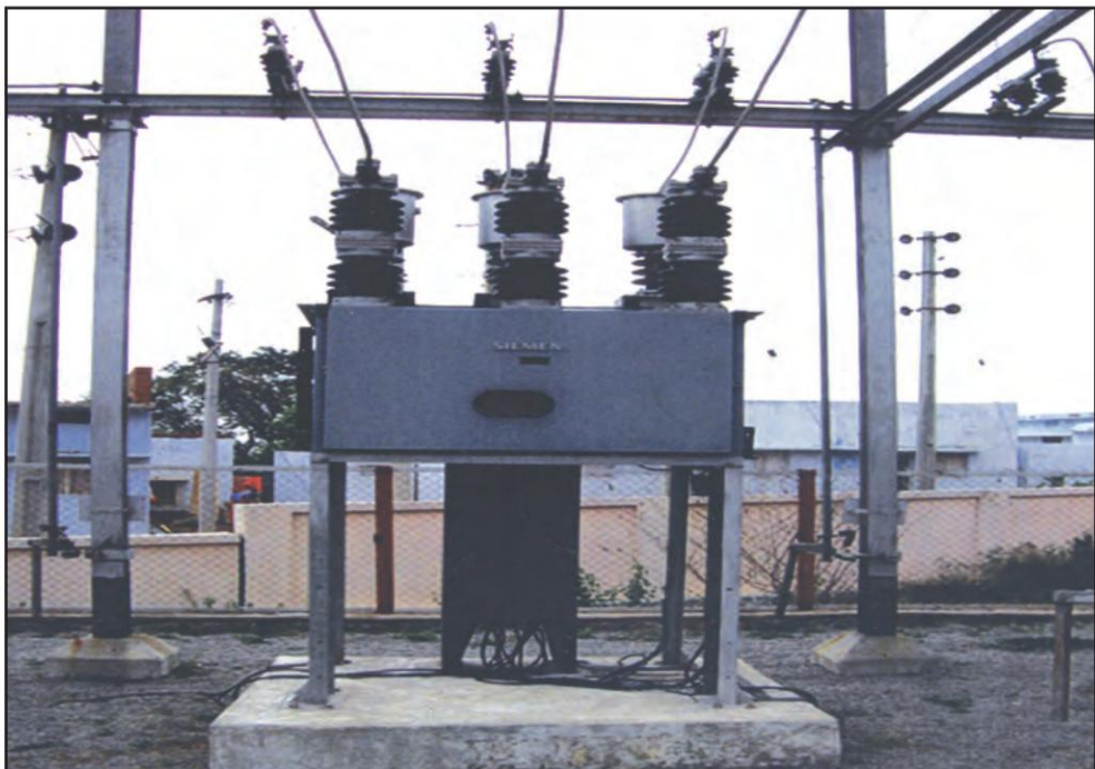
Plate 9 11 KV feeder control and metering cubicle
