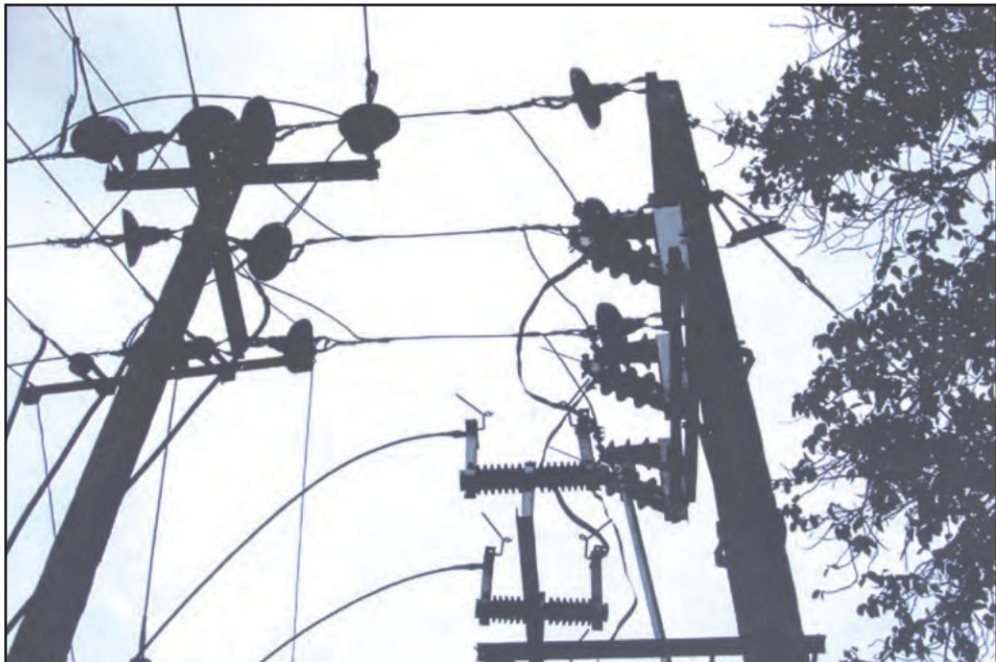
Plate 2 11 KV Isolator switch and surge diverter, Horn gap fuse mounting for the substation in Plate 1
