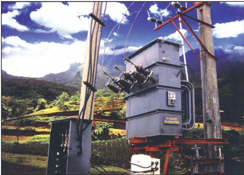
Plate 1 Pole mounted substation 11,000 V/415V
