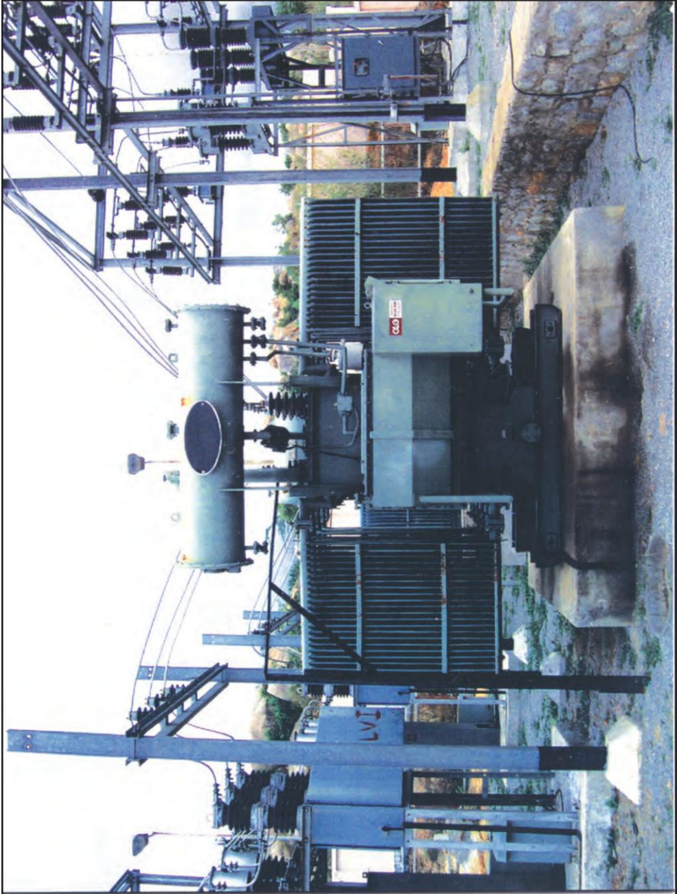
Plate 7 33/11 KV Power transformer (5MVA)
