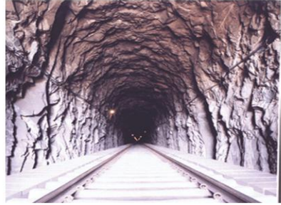
(b) Bhatan tunnel, Mumbai-Pune Express way
