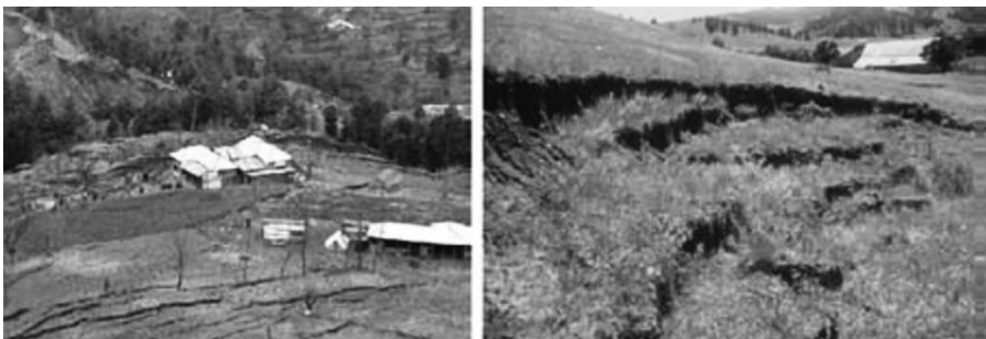
Fig. 12.4 Cracks on the ground surface indicating initial process of creeping
