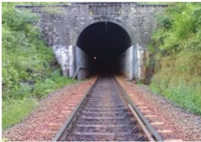
(c) Karbude tunnel, Maharashtra
