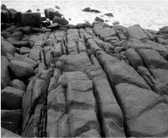
Fig. 8.21 Sheet joints in granite
