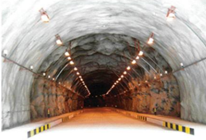
(a) Jawahar tunnel, Kashmir
