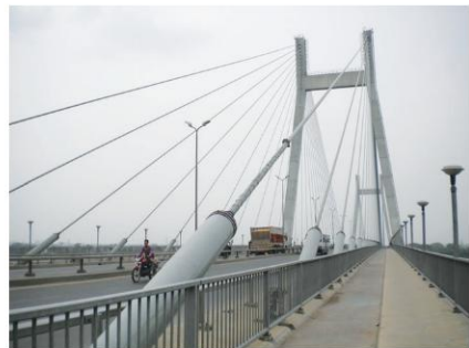
(f) Naini Bridge, Allahabad
