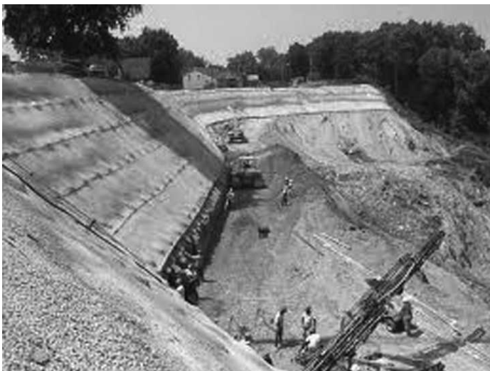
Fig. 12.6 Slope modification and stone pitching
