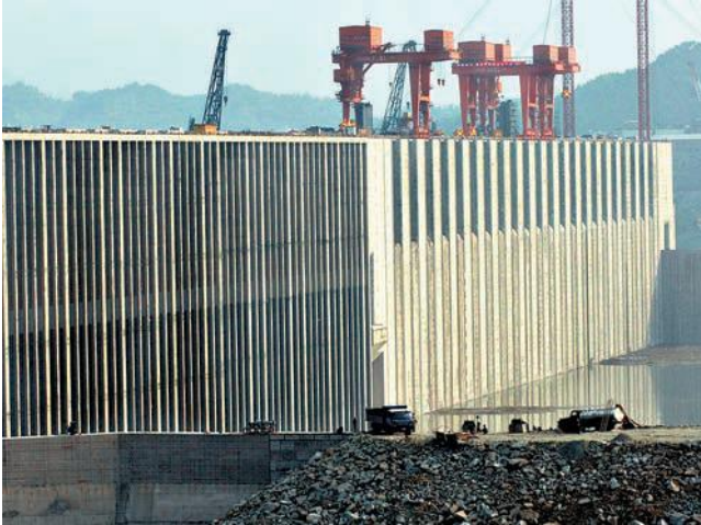
Large trucks are dwarfed by the 185-meter-high sluice gates of the Three Gorges Dam. China began filling the reservoir in a major step toward completion of the world's largest hydroelectric project. The level is expected to reach 135 meters (446 feet), inundating thousands of acres, including cities and farms along the Yangtze. (AP/Wide World Photos)
