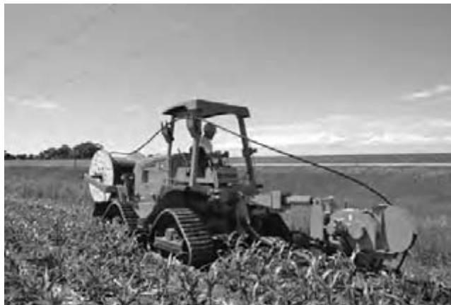
Fig. 1.12 Plowing operation for direct burial of optical fiber cables. (Photo © VERMEER CORPORATION. All Rights Reserved; www.vermeer.com .)
