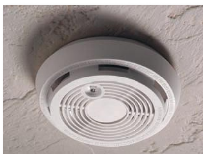
Americium-241 is a radioactive element contained in smoke detectors. The decay of \alpha particles creates an electric current that is interrupted when smoke enters the detector, sounding an alarm.
