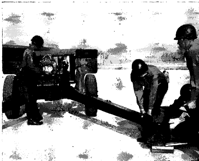
Figure 46. Blocking trail to level trunnions for bore sighting with gunner's quadrant atop breech ring.
