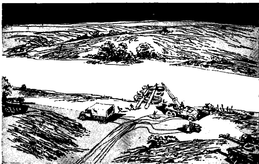
Figure 128. (Added) The use of 18-inch searchlights in the general illumination role to facilitate bridge construction work.
