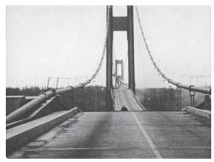
**FIGURE 13.1 The collapse of the Tacoma Narrows Bridge.** The dramatic collapse of the bridge was captured on film, and some of the footage is available in video files.
