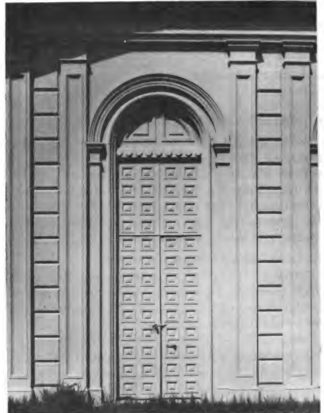
Figure 10. Door of cast-iron Storehouse at Watervliet Arsenal.
