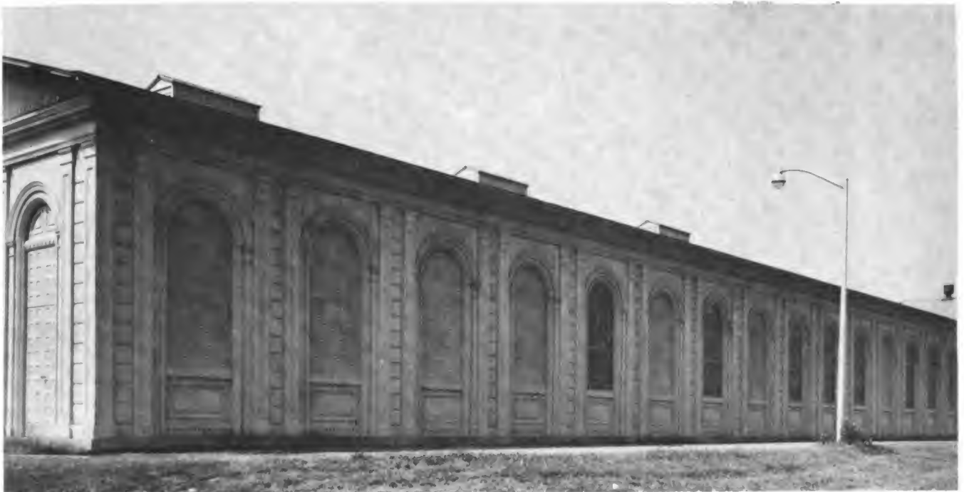
Figure 11. Example of Category II: Storehouse of cast-iron at Watervliet Arsenal.
