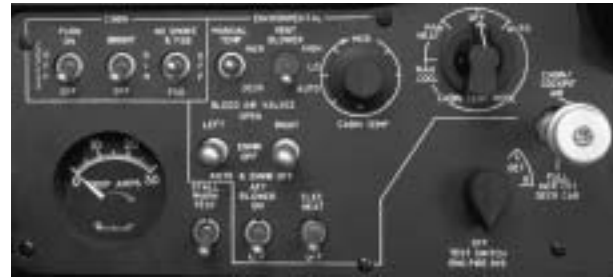
Figure 1-5. Cabin Lights Control Switch (BB-1439, 1444 and After)
