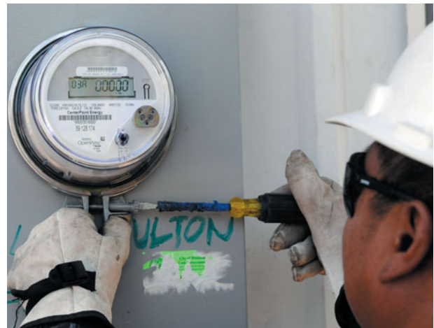
A smart meter being installed
