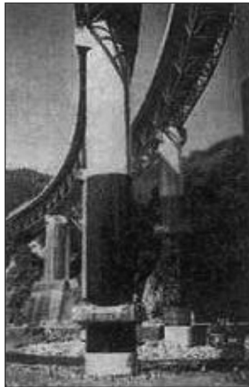
Figure 3.7. Fiber-sheet jacketing of high-pier.
