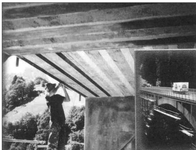
Figure 3.13. Strengthening of the Tanberg Bridge, Austria.
