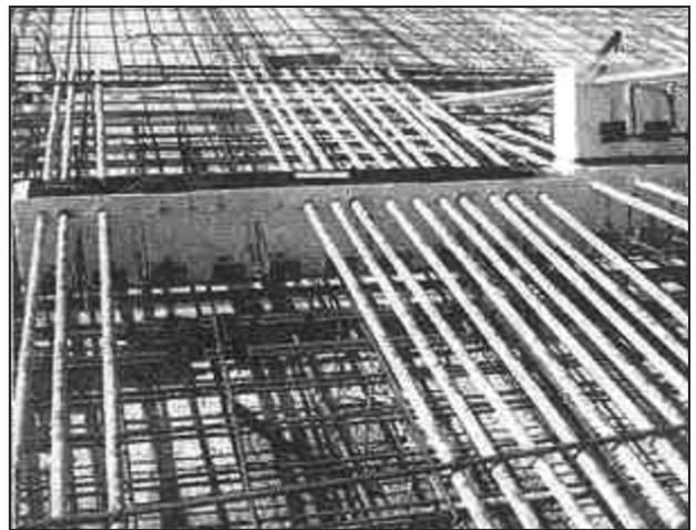
Figure 3.9. Thermal insulating element.
