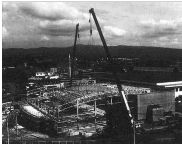
Figure 3.5. FRP truss structure for roof of pool.
