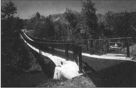
Figure 3.3. Stress-ribbon bridge.
