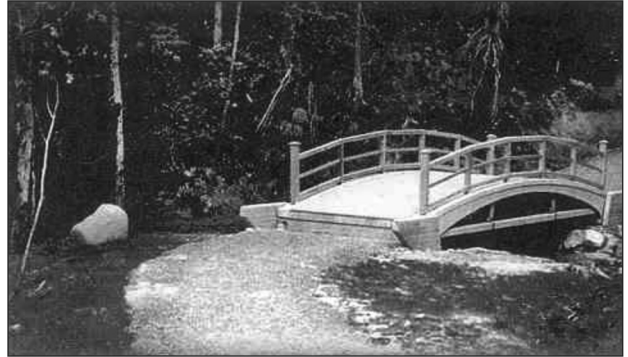
Figure 3.8. Oppegaard Footbridge near Oslo, Norway.
