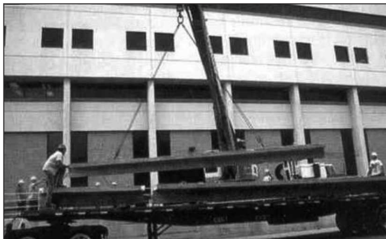
Figure 3.17. Shipping of test specimen of FHWA research program to the University of Wyoming.
