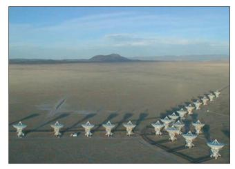
of such arrays to tens of kilometers. The workhorse of contemporary radio astronomy is the Very Large Array (VLA) in western New Mexico. The VLA, shown in Figure 6.41, consists of a Y-shaped configuration of 27 dishes that can be moved on railroad tracks to span a region as large as 40 km across. Astronomers from around the world use the VLA to map radio objects with a resolution of about 1 second of arc. This resolution compares favorably with that of ground-based optical telescopes.
